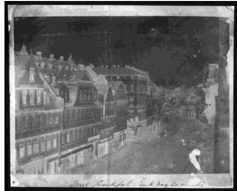
Figure 7: same image as figure 4, recto, viewed with transmitted light, after treatment.
